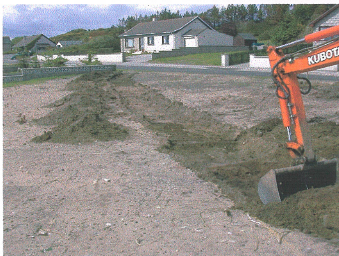
5. Area A. Footpath, topsoil stripping to a depth of 10-15cm, view from east.
