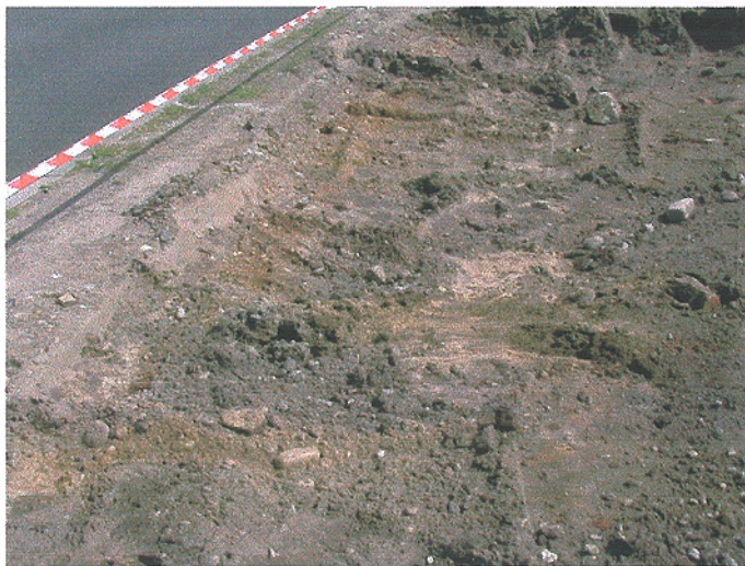
4. Layby, Area A. Lighter sand indicating the possible natural surface at a depth of 0.3m
