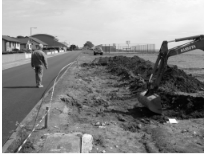
3. Layby, Area A. Stripping of topsoil to a depth of 0.3m, view from SW
