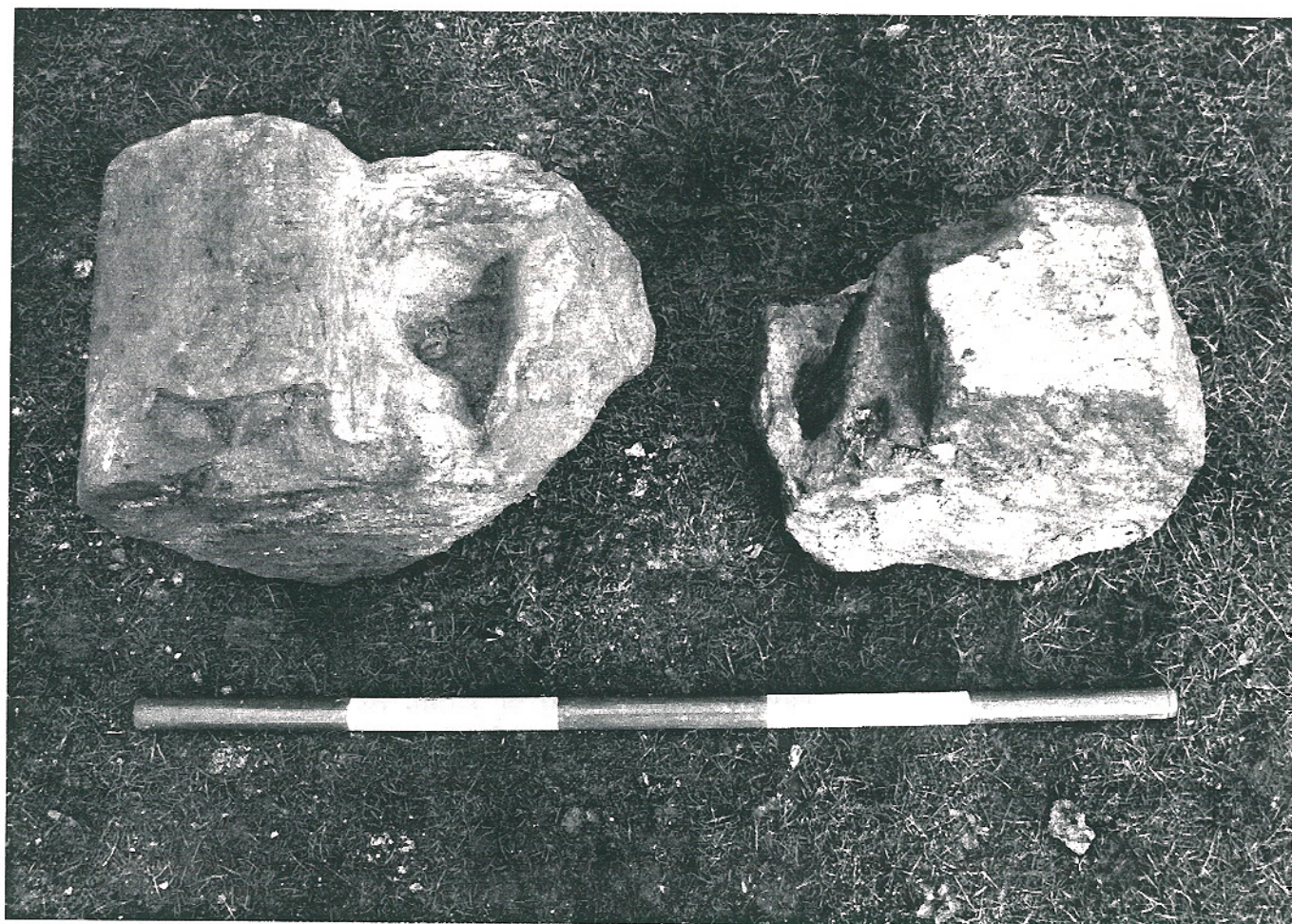
Figure 14. Photo of window jambs from tower with sockets for iron grills.
