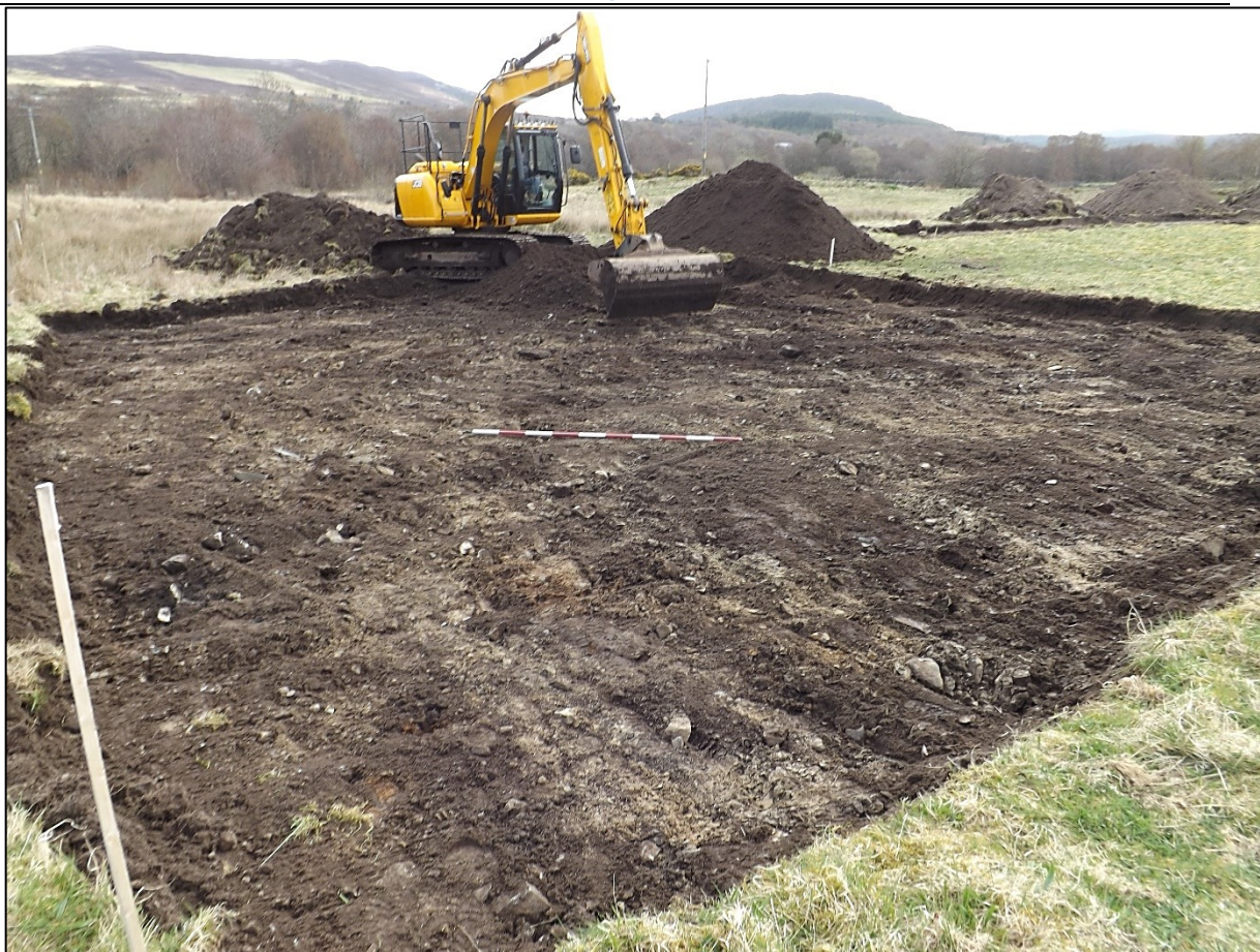
Figure 9 - Topsoil stripping of the garage/workshop area nearing completion. Facing NE. Scale 2m.
