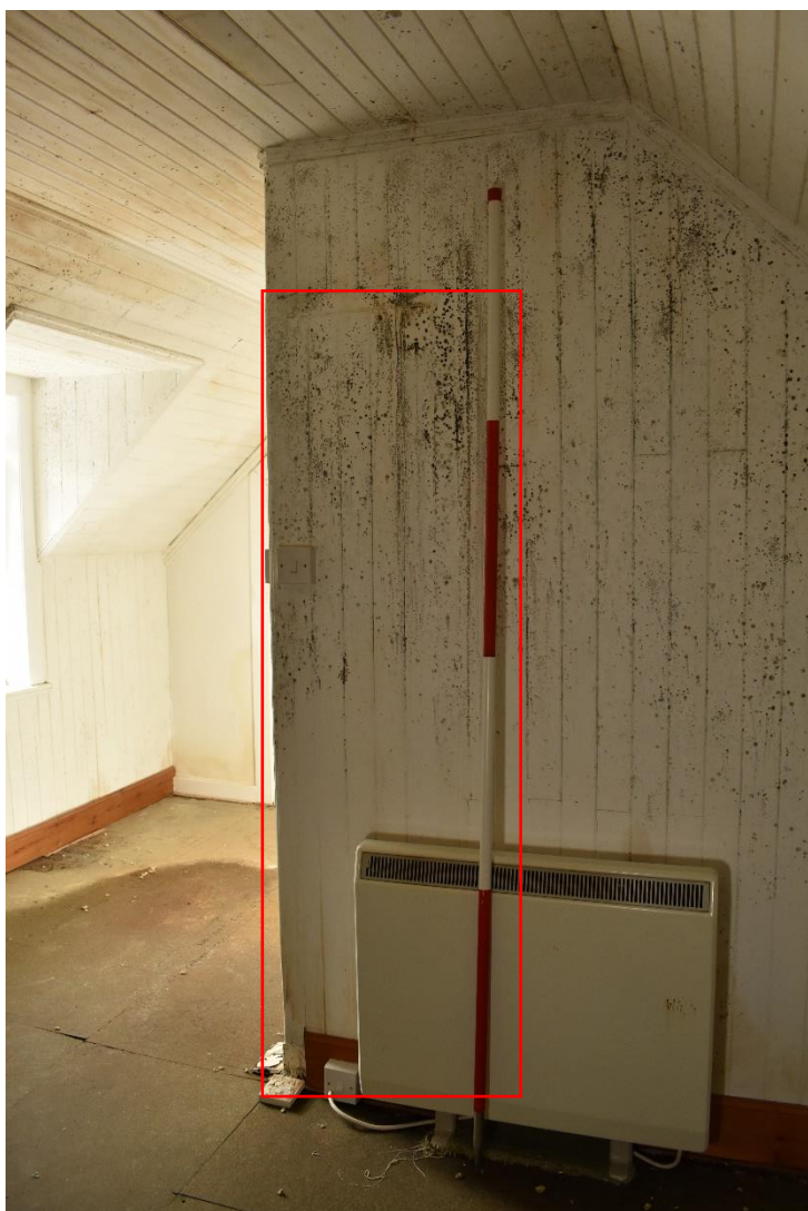
Figure 33: Evidence of blocked doorway in eastern wall of FF4
