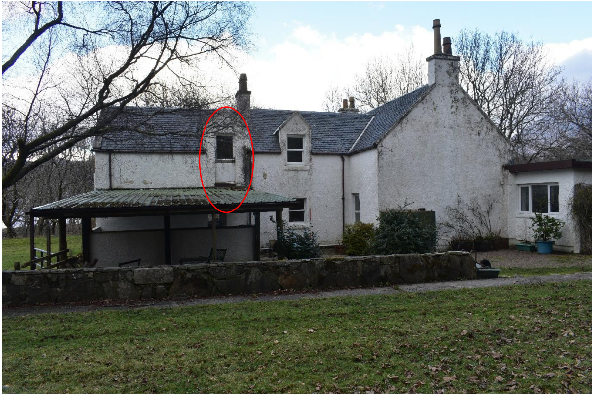
Figure 10: View of Roshven Farmhouse southern elevation showing what appears to be a blocked door in one of the dormer windows (W21) outlined in red.
