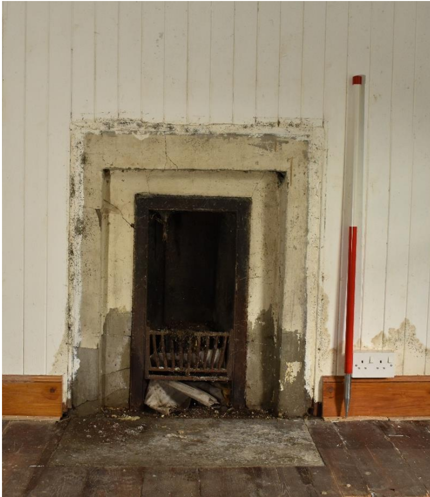
Figure 31: Evidence of cast concrete fireplace in room FF2.
