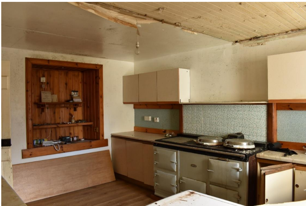
Figure 18: Room GF10 with shelf built into a blocked window opening in the eastern wall
