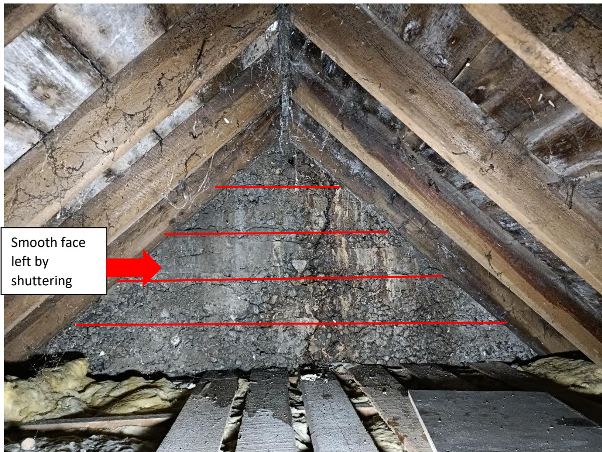
Figure 30: Evidence of concrete construction with “lifts” and evidence for the use of shuttering can be seen in the gable wall of the southern elevation.
