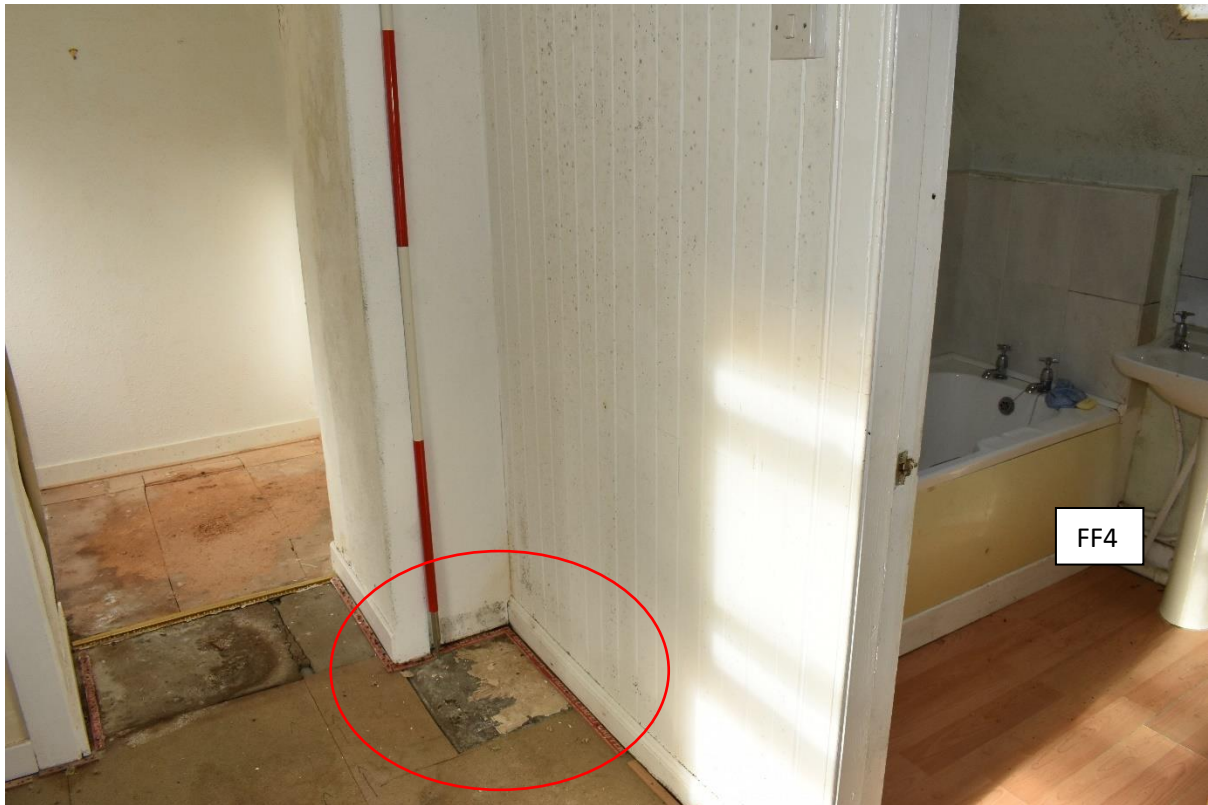
Figure 21: Detail of remains of a concrete hearth which continues underneath the southern wall of FF4
