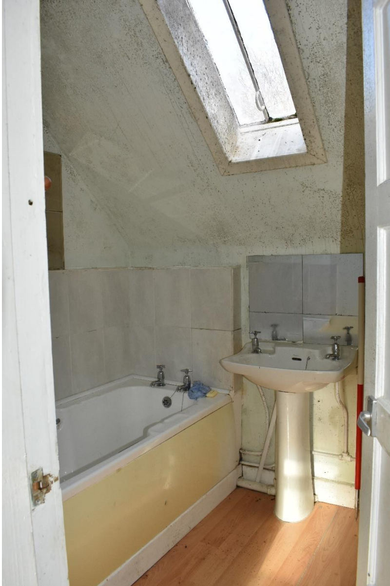
Figure 24: Room FF4 with cast iron roof light
