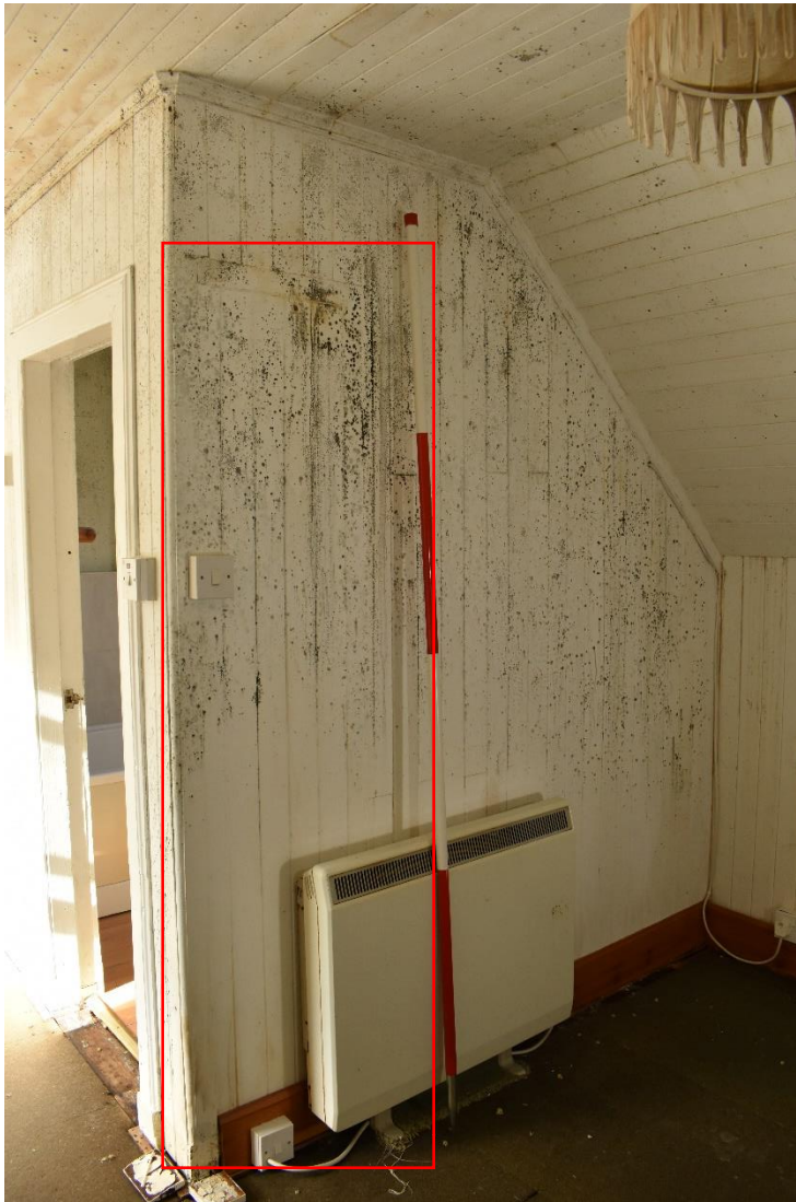
Figure 20: Evidence of blocked door opening in wall of Room FF4
