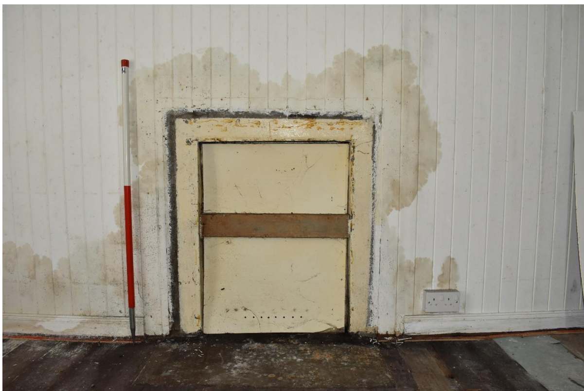
Figure 23: Fireplace and detail of concrete surround and hearth room FF3
