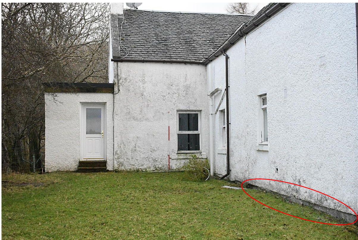
Figure 35: Block work footings of later rear extension indicated in red
