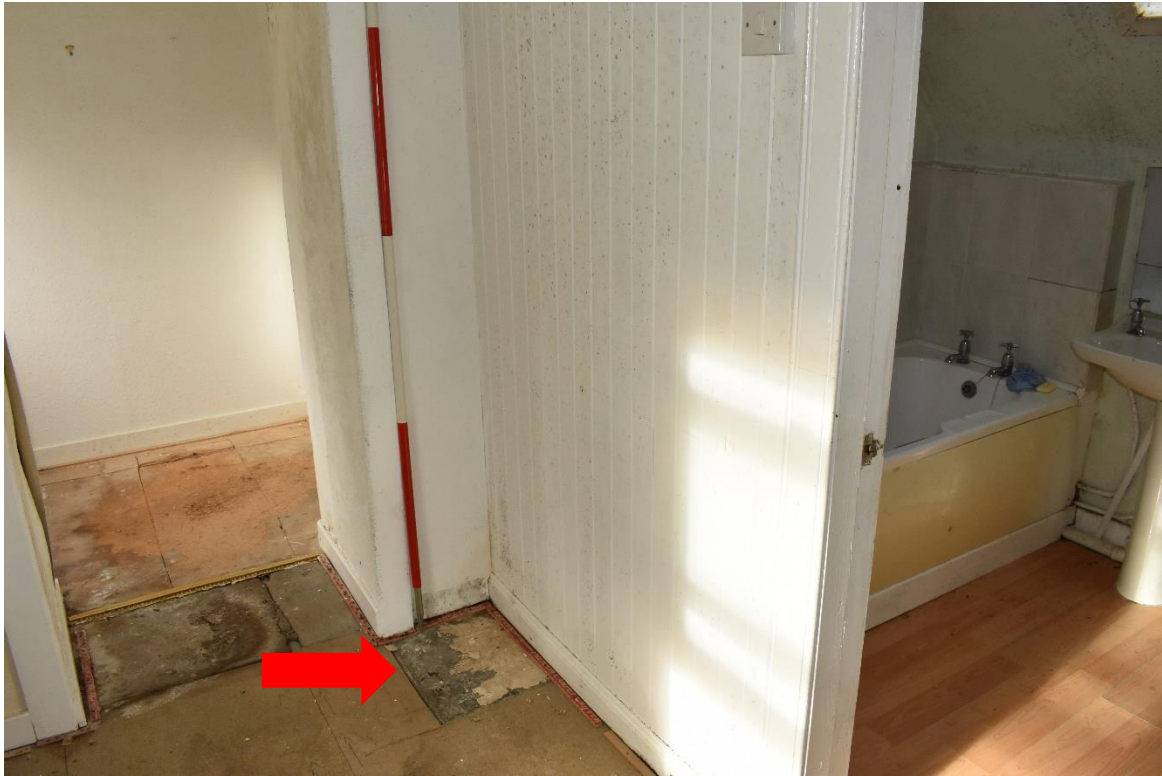
Figure 34: Evidence of hearth stone (feature F1) continuing under wall of bathroom FF4
