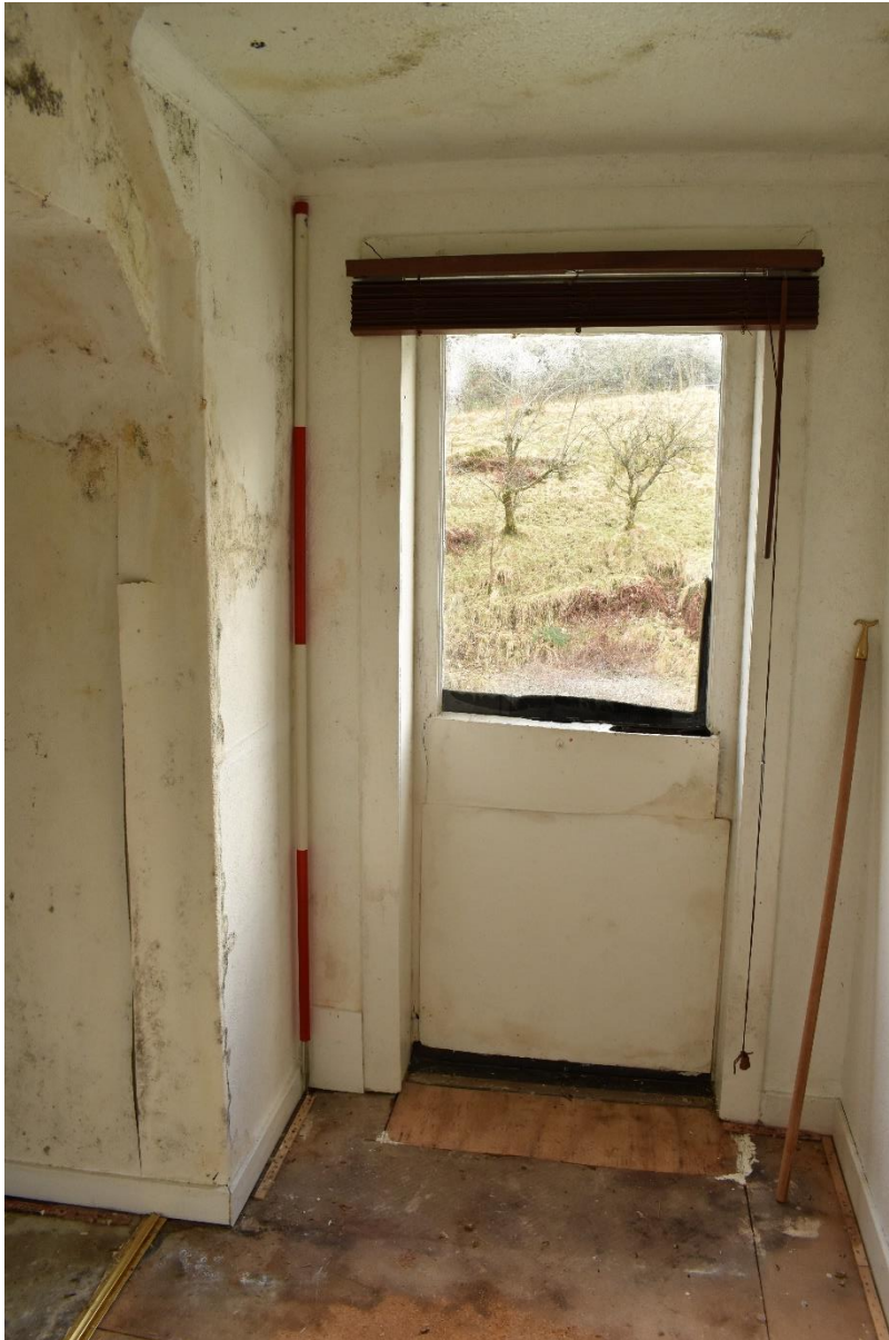
Figure 25: W21 Doorway inserted into the dormer window opening and then partially blocked (note threshold)
