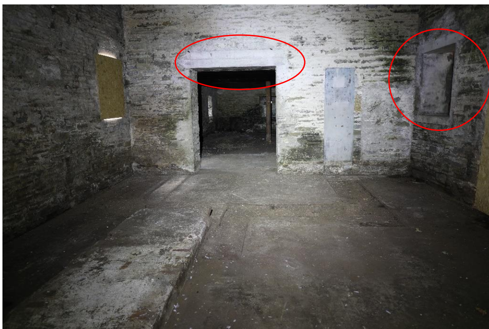
Figure 29: Grain Store 2 showing channels and fixing points in floor (alterations to openings highlighted)
