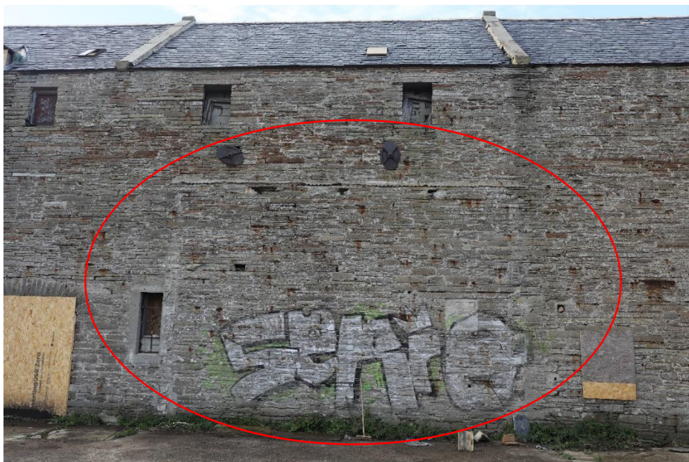
Figure 27: Evidence of former extension to eastern elevation
