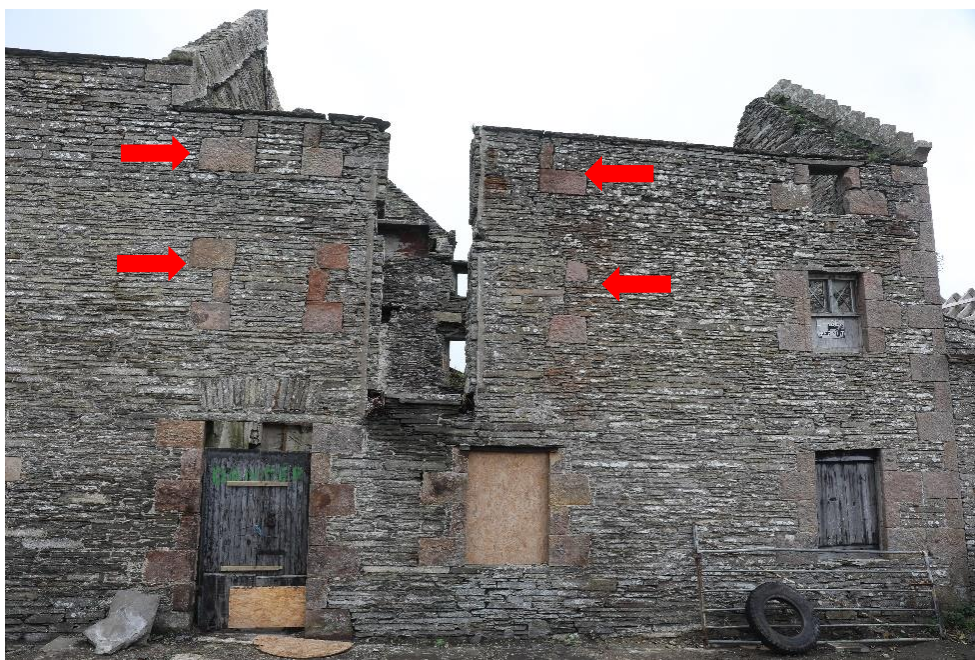
Figure 42: Building break left by insertion of Chute 2 into Drying Kiln 1 with evidence of red sandstone margins from previous windows
