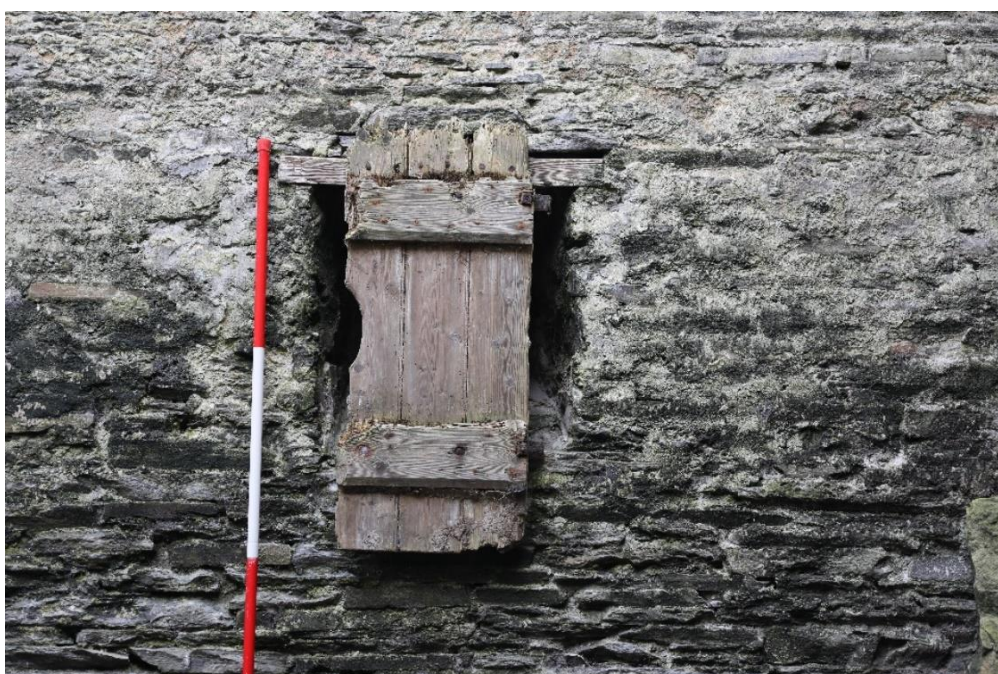
Figure 13: Remains of a shutter to ground floor window W3.
