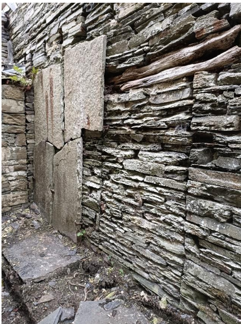
Figure 20: Detail of internal wall of wheel-house with earlier blocked windows and Caithness Flagstone lining
