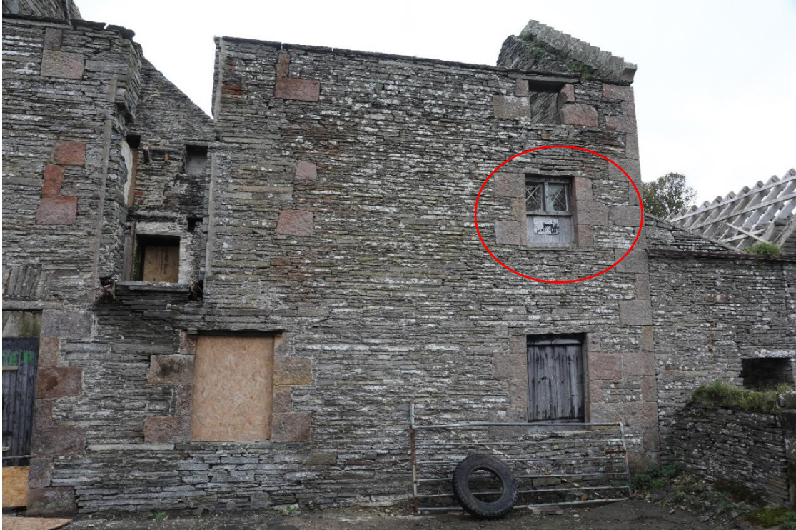
Figure 9: Unusual window with cross shaped glazing bars in westernmost bay of original c.1818 range.
