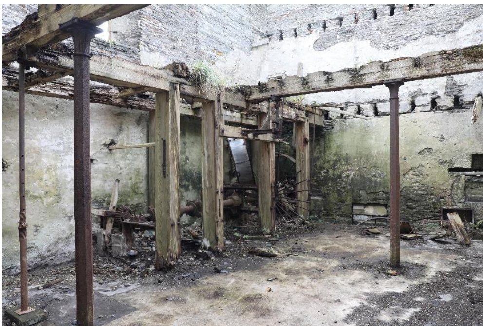
Figure 16: General view of remaining mill workings
