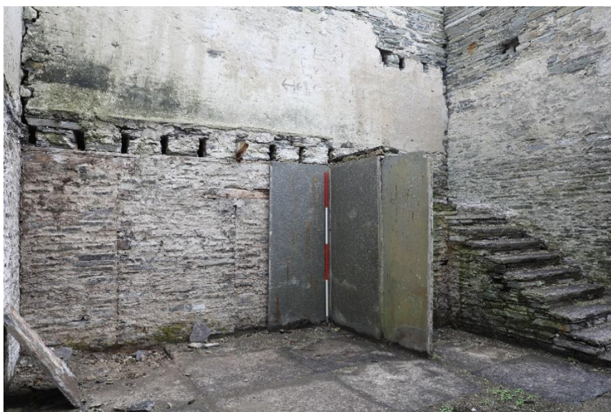
Figure 40: Western wall of Grain Store 1 showing blocked door openings with the right hand side one being partial obscured by the later Caithness Flagstone structure
