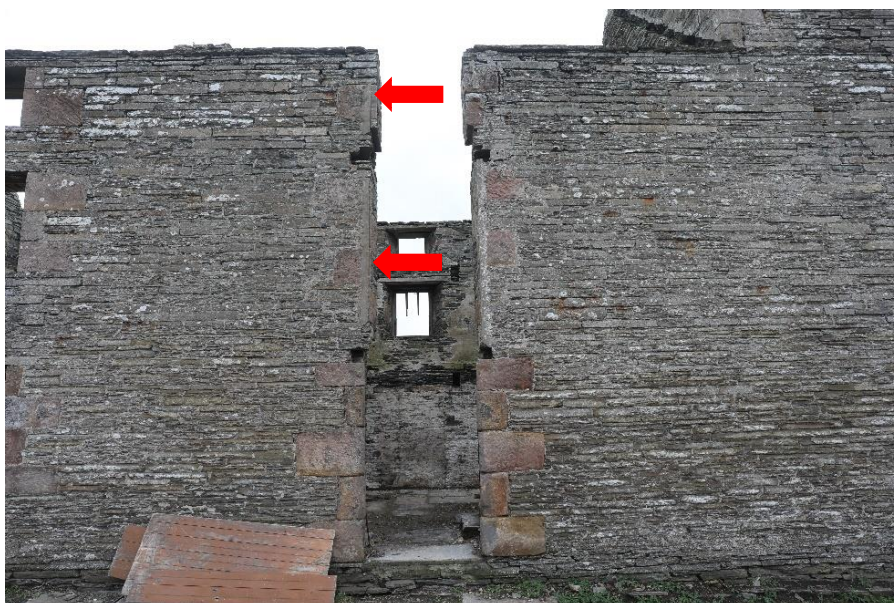
Figure 41: Building break left by insertion of Chute 1 into Drying Kiln 1 with evidence of red sandstone margins from previous windows
