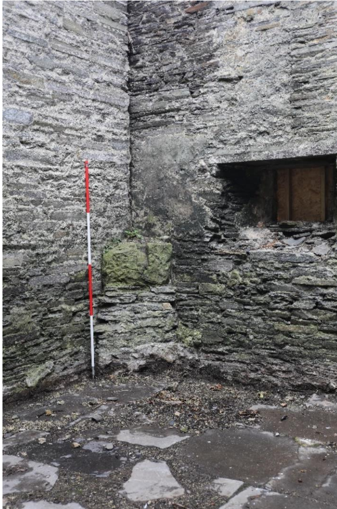
Figure 14: Detail of stone pillar with carved angled socket
