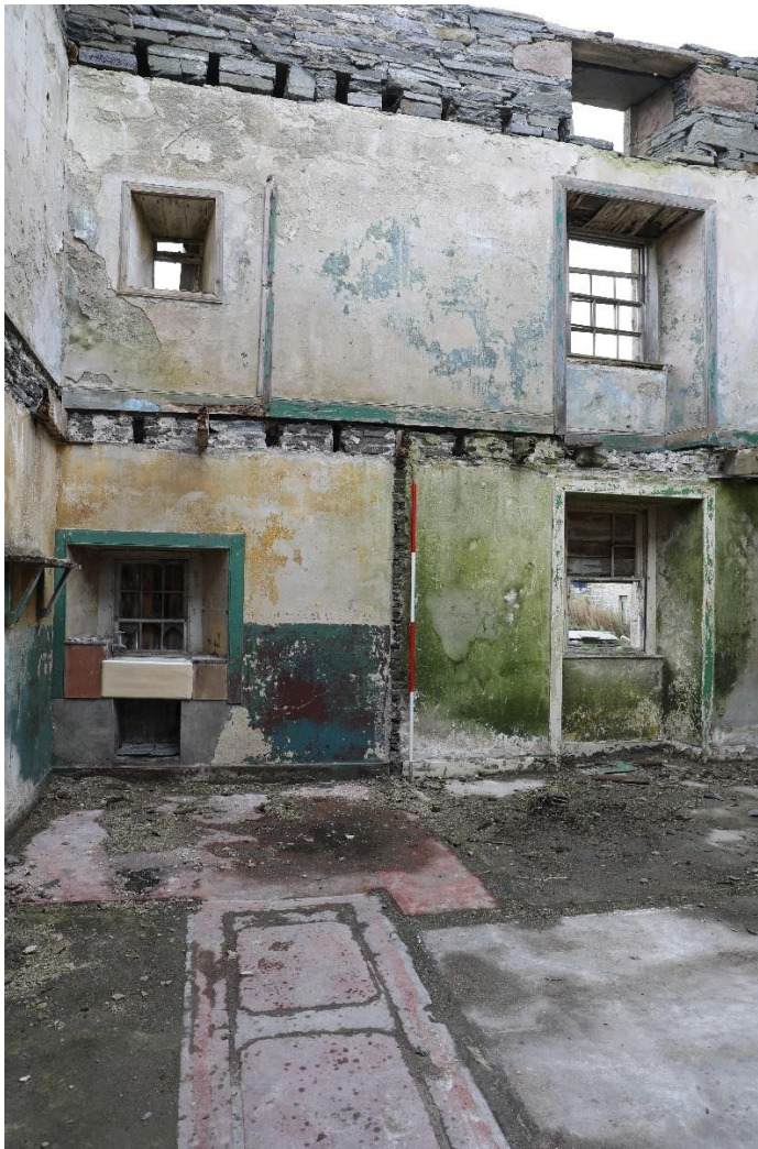
Figure 10: Photograph showing evidence of internal partitions surviving in the floor surface of the Miller's House.
