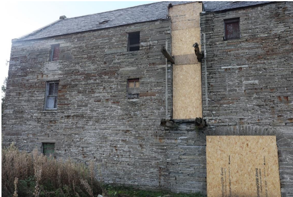
Figure 24: Remains of chute or sack hoist
