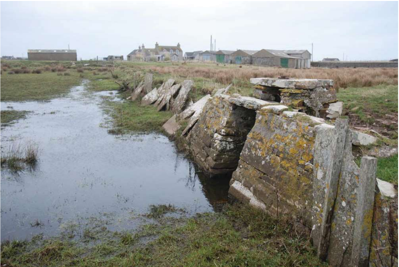
Plate 95: The mill pond, detail of the opening to the east side of the north wall of the mill pond for the mill lade, from the east
