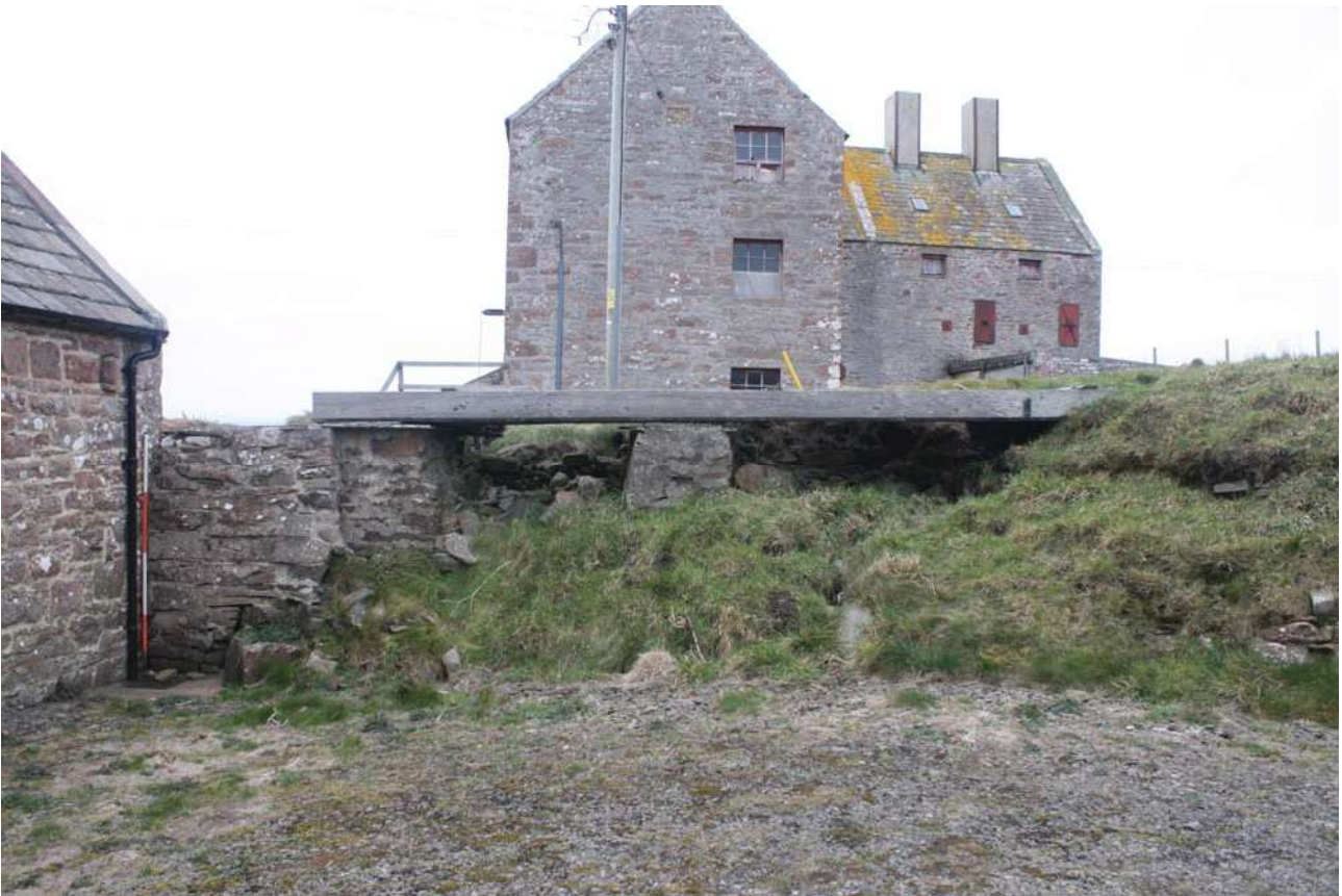
Plate 107: The timber mill lade, general view of the southernmost east/west lade showing the stone buttresses supporting it, from the south
