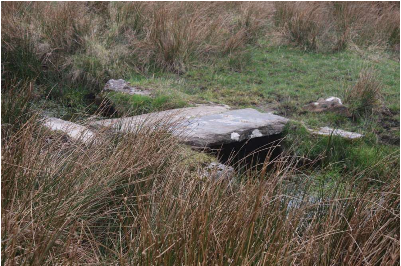
Plate 100: The mill lade, detail of the small capstone over the lead just to the south of the road, from the north-east
