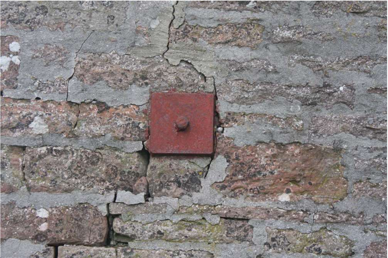
Plate 11: The mill, detail of the square building tie in the east elevation, from the east
