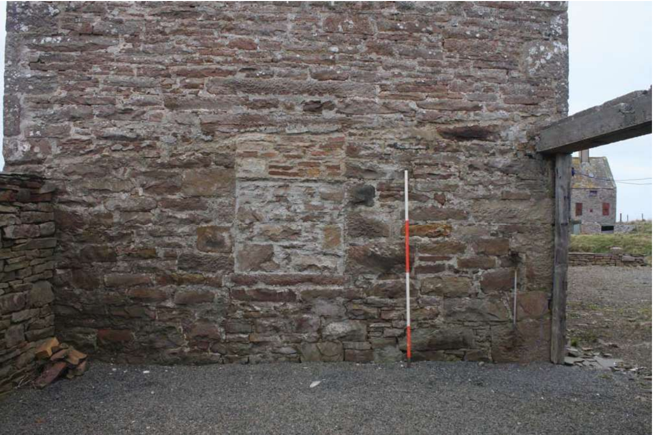
Plate 119: The southernmost mill cottage, detail of the stone-blocked window on the south elevation from the south
