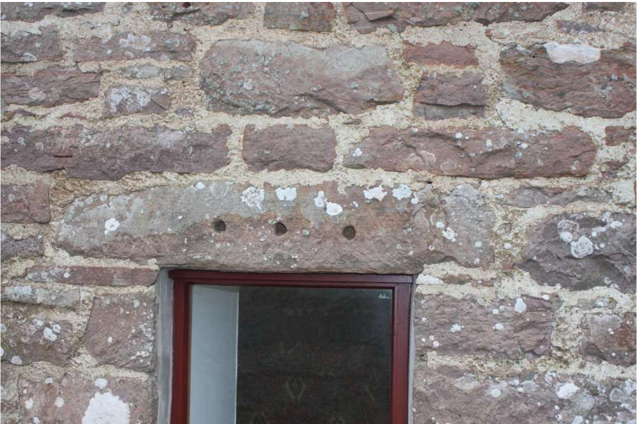
Plate 110: The northernmost mill cottage, detail of the holes in the lintel of the northernmost window on the east elevation, from the east
