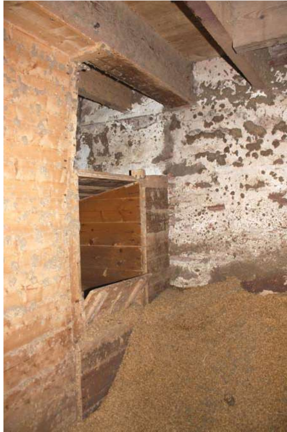
Plate 43: The mill, Room 0/2, detail of the west side of the south wall of the husk cupboard showing the timber chute from the winnowing machine within, from the north-east
