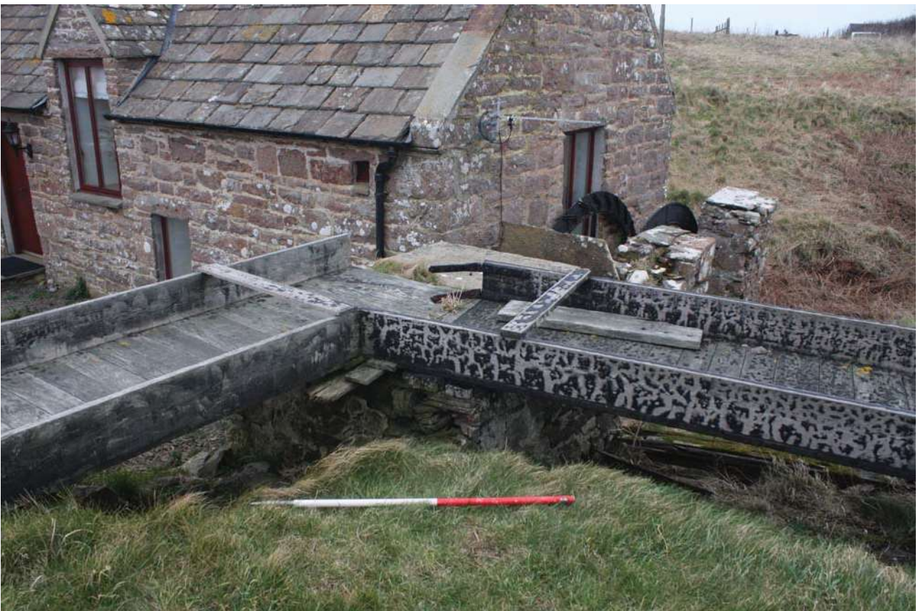
Plate 106: The timber mill lade, detail of the corner between the two lades, from the north-east - note the hinges for the former sluice gate
