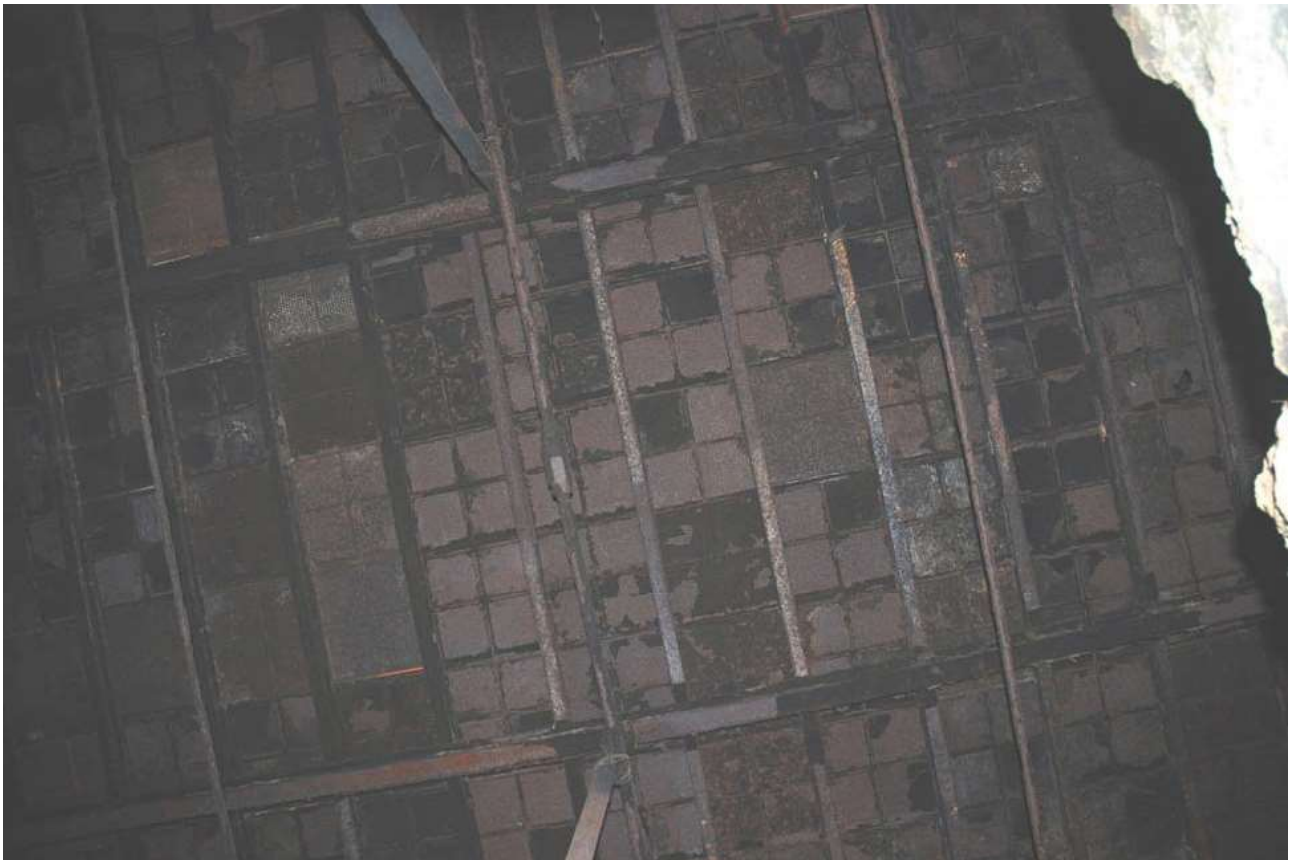
Plate 50: The mill, Room 0/4, general view of the underside of the drying floor looking up from the base of the furnace
