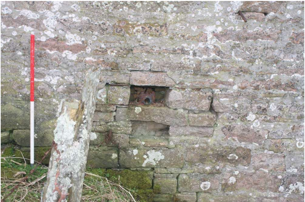
Plate 24: The mill, detail of the small chute and bearing block to the base of the north elevation of the mill on the west side, from the north
