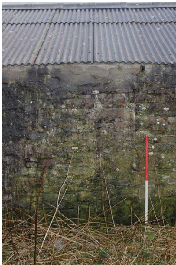
Plate 128: The northernmost abandoned mill cottage, detail of blocked door in the north elevation from the north
