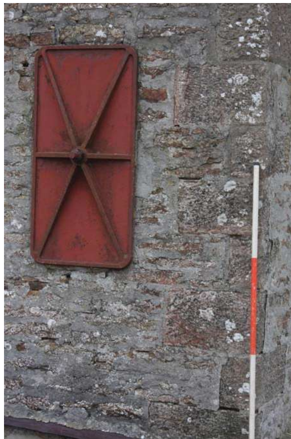
Plate 16: The mill, detail of the easternmost large rectangular building tie on the south elevation of the kiln, from the south-east
