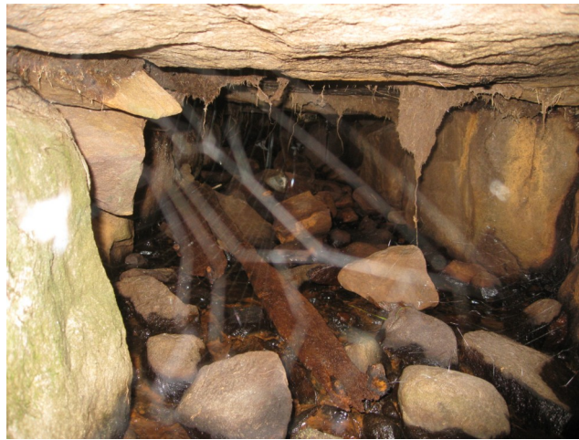
64 NG 74929 71292 30m Stone bridge width 4m
