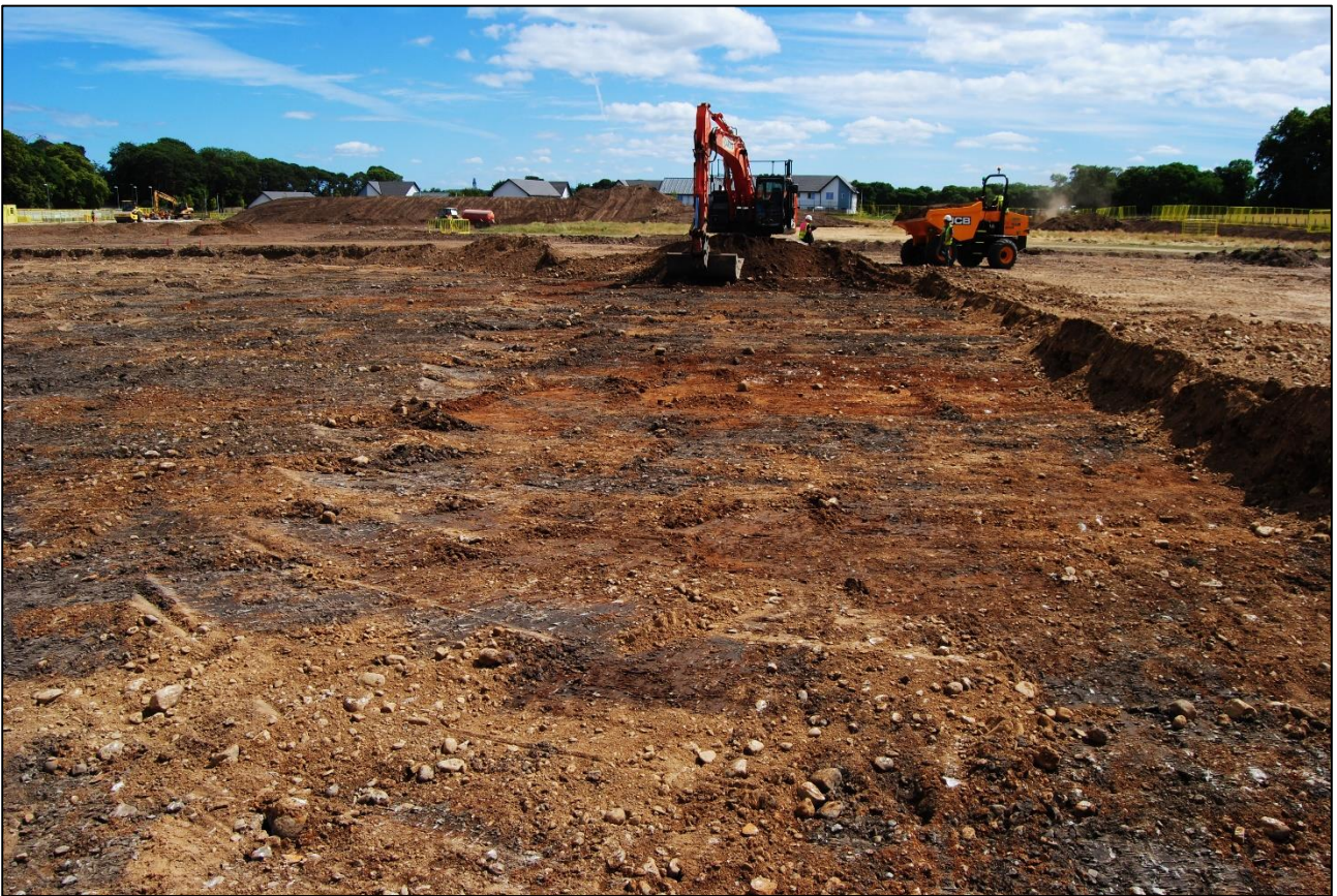
Plate 4: Stripping an area of made ground, facing SE
