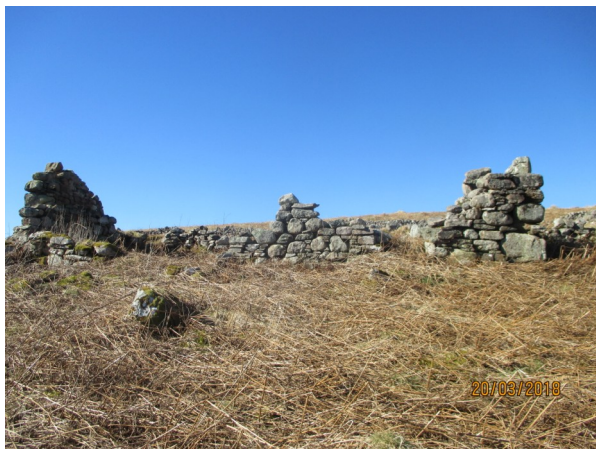
The house, note the layered stones in walls
