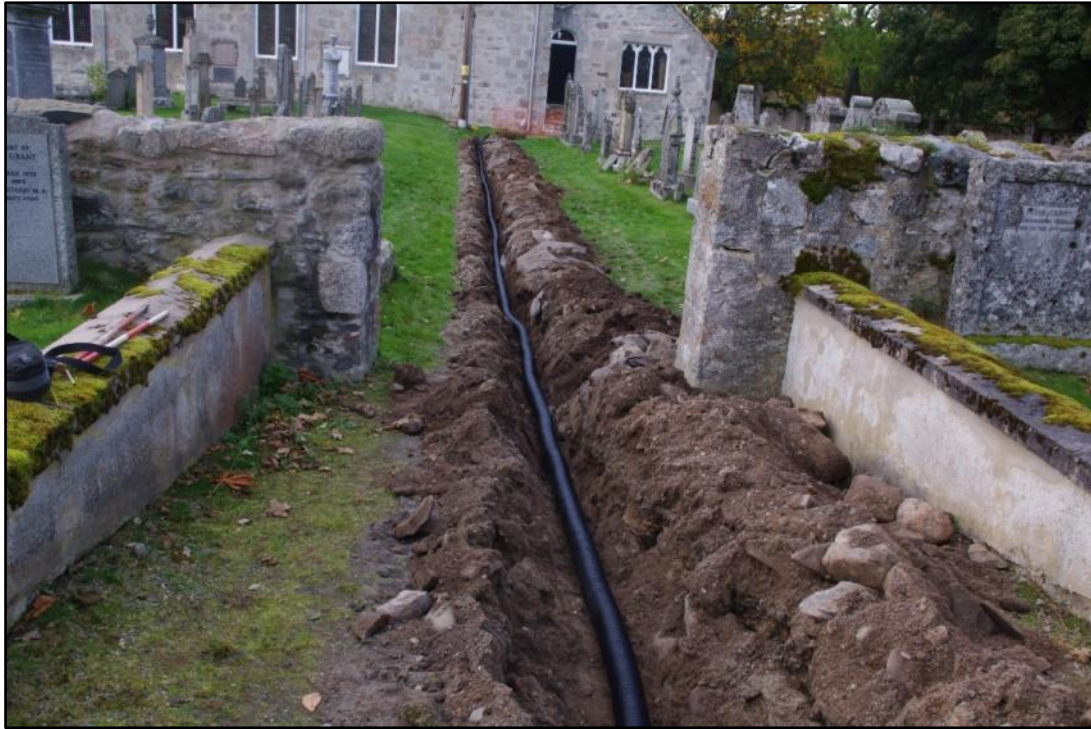
Photograph 3: The cable trench through the churchyard with ducting installed
