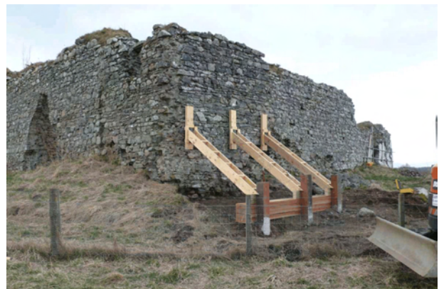
Plate 5 Intervention 5 showing temporary supports
