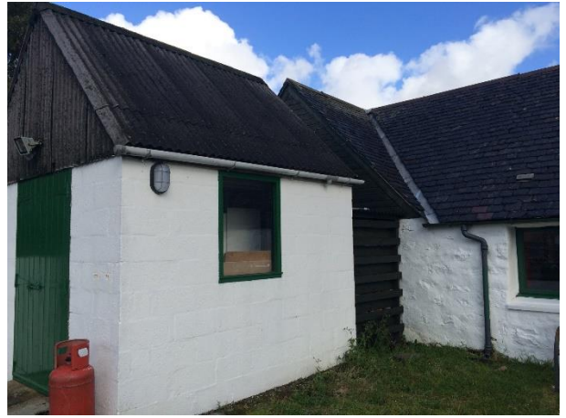
Store - corrugated roof and painted block work walls
