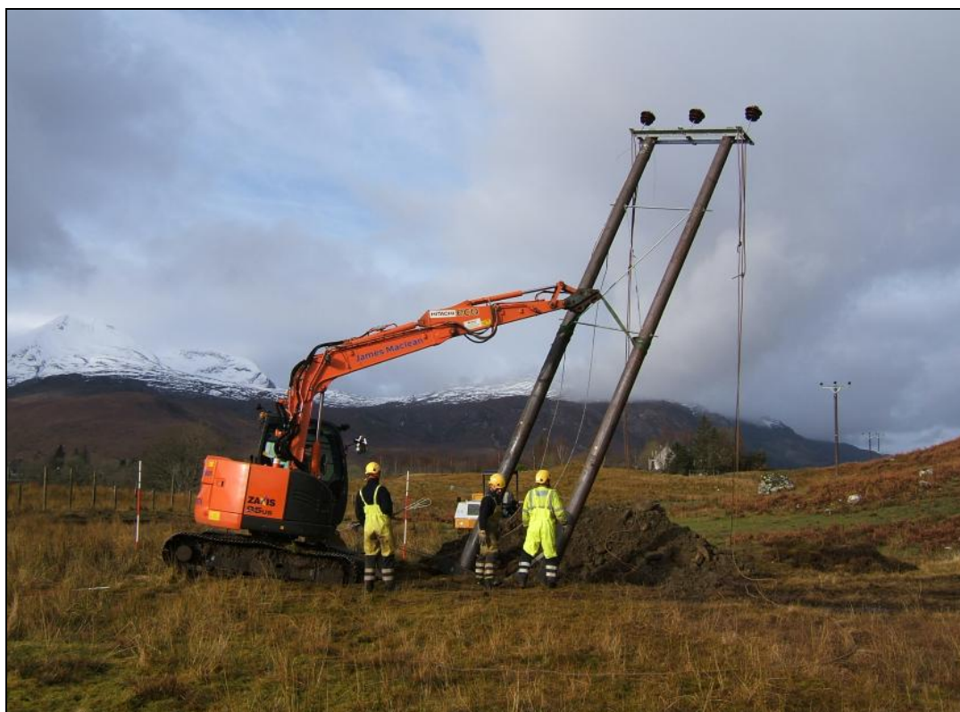
Lifting Pole 113 into position, viewed from the east
