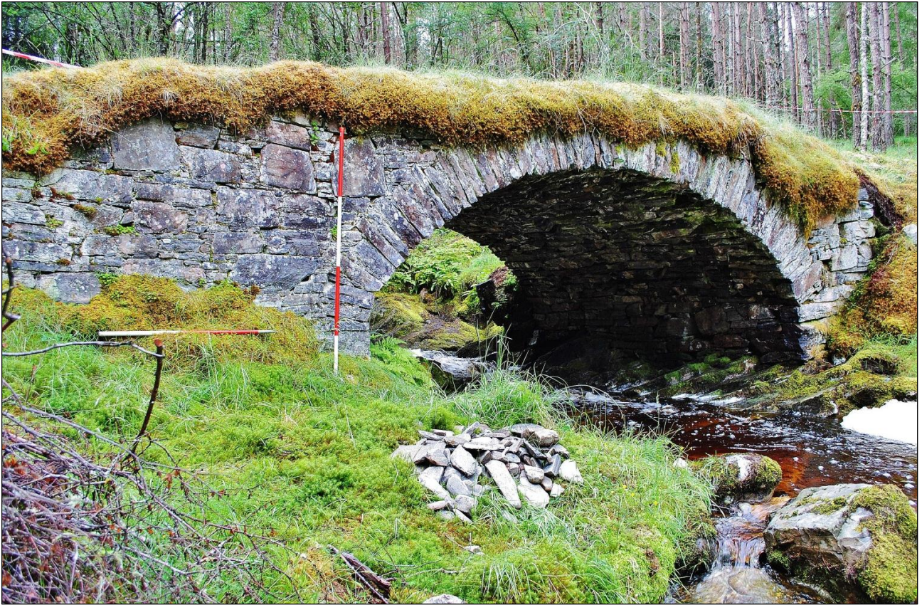
Plate 1 North arch of bridge, pre-conservation, showing eastern abutment, facing SW (CP7)
