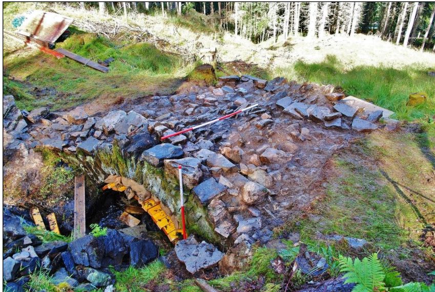
Plate 6 Pre-conservation image of SSW arch / parapet and voussiers, facing NNW (CP16)
