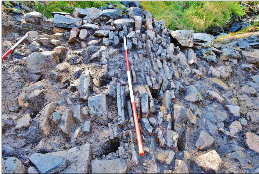
Plate 5 Pre-conservation image of bridge surface and voussiers, facing SSW (CP15)
