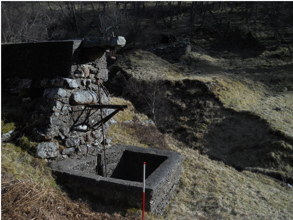
Plate 4 – Sluice-gate housing Site 16b and the tiered back edge of the dam Site 16c
