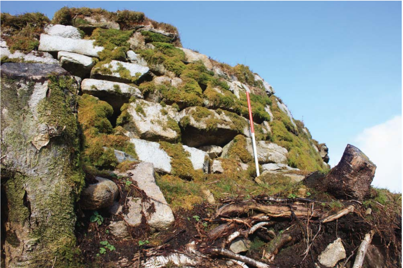
Plate 11: Missing blocks in the outer wall face at Point E, facing NE
