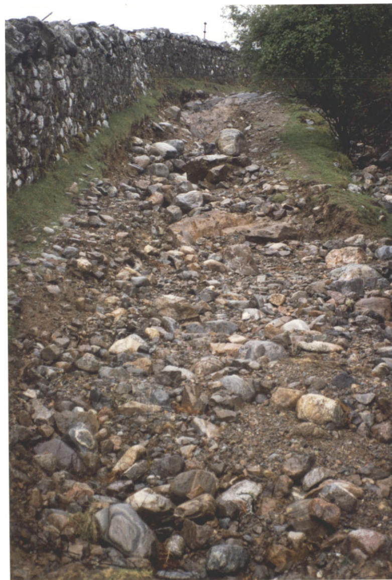
10. Washed out surface with bedrock showing. Ch. 230.
