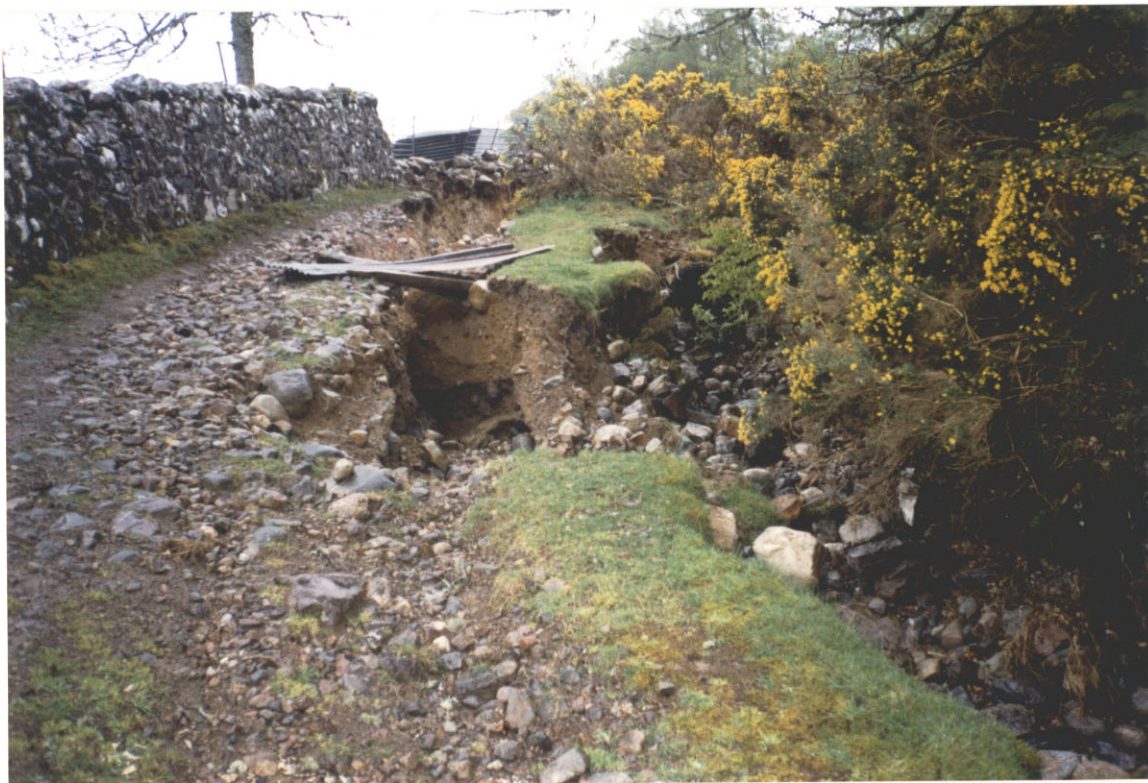
5. Ruts and ditch, at Ch. 130, looking uphill to collapsed wall.
