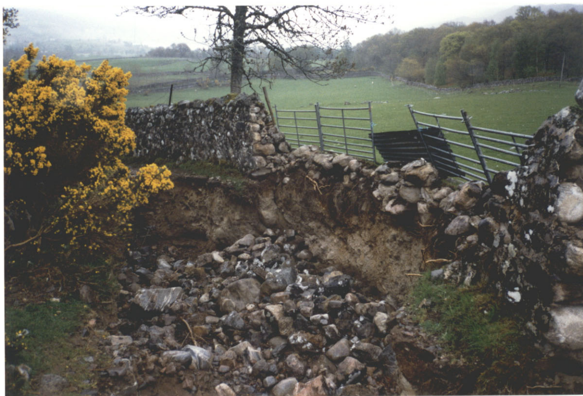
6. Collapsed wall at Ch. 150, looking downhill.
