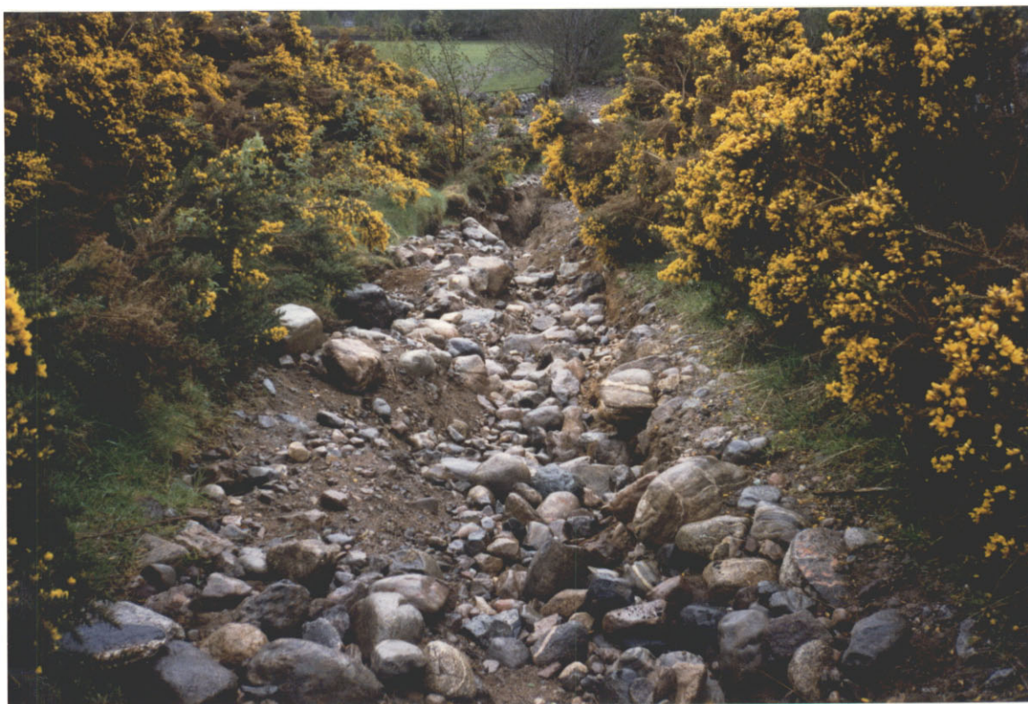
1. Looking downhill to public road. Showing road surface washed away and start of deep ruts.
