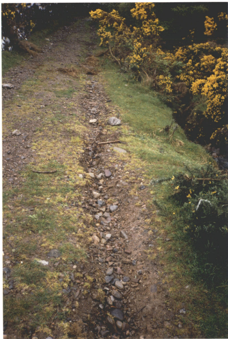
·3. Existing road surface with minor rutting. Ch 70
