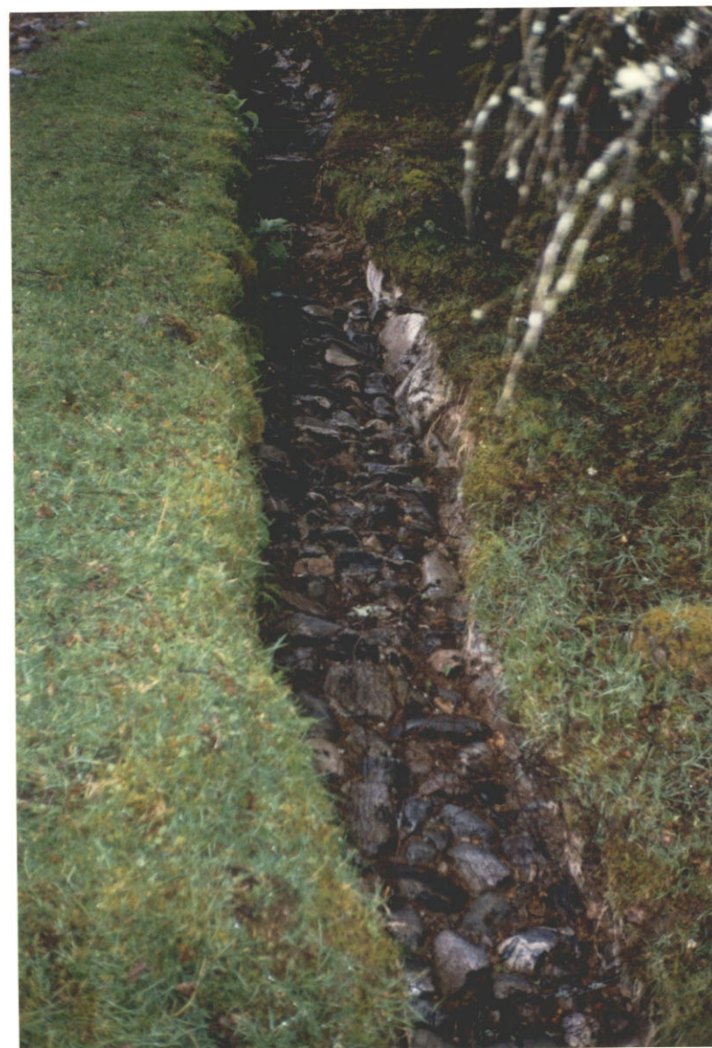
·4. Paved ditch in good condition. Ch. 90
