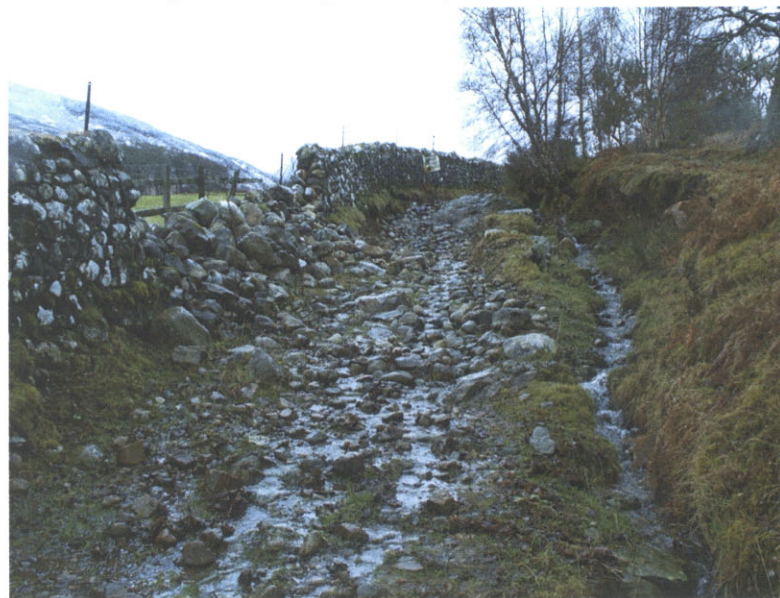
CH210 –rutting and wall collapse (see old photo9)
