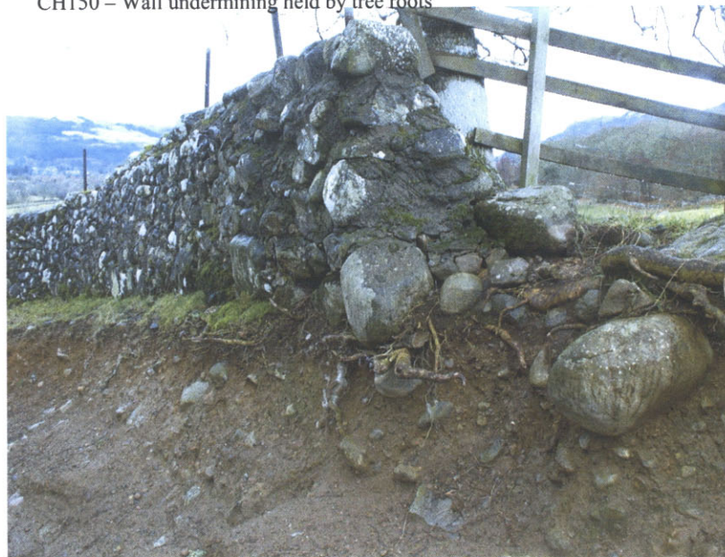
CH150 – Wall undermining held by tree roots
