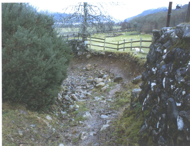
CH170 Washout and wall collapse (see old photo 6)
