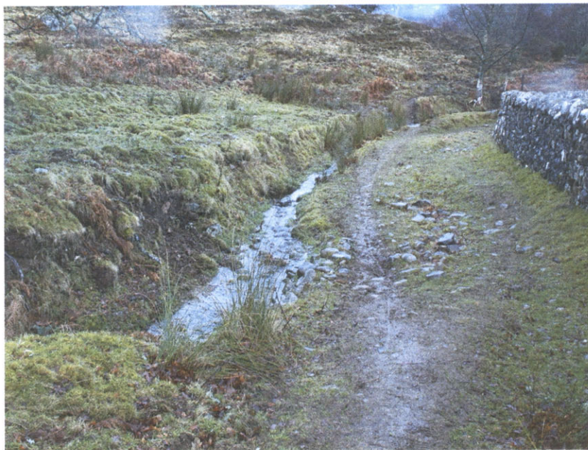
CH330 – Stream cutting cutting into path
