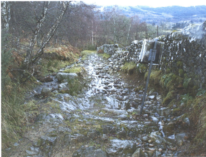
CH270 – Rock outcrop and wall collapse
