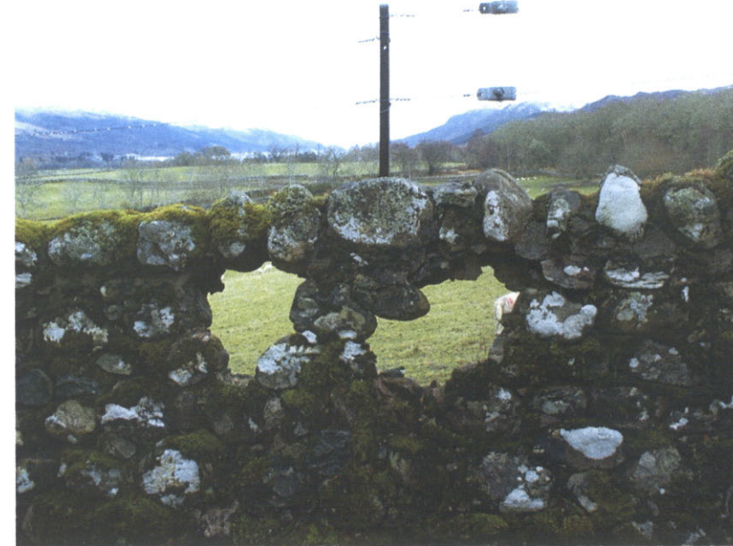
CH110 – wall collapse on field side
