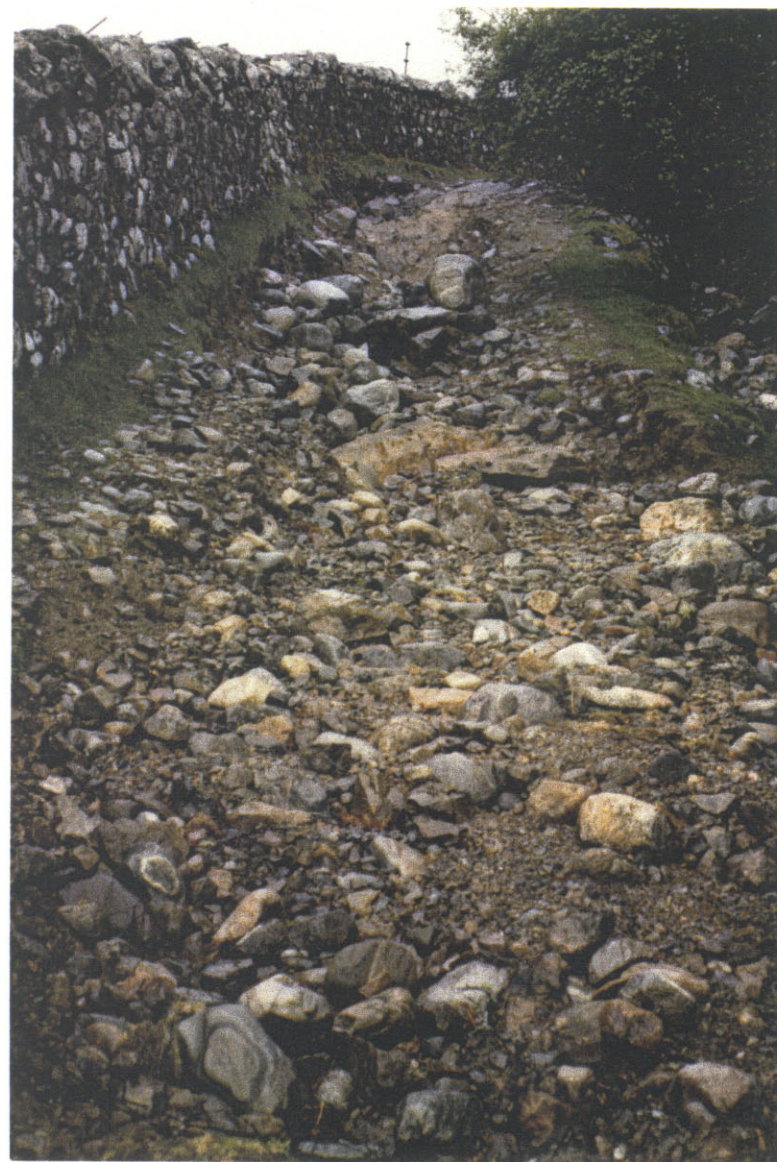
10. Washed out surface with bedrock showing. Ch. 230.
