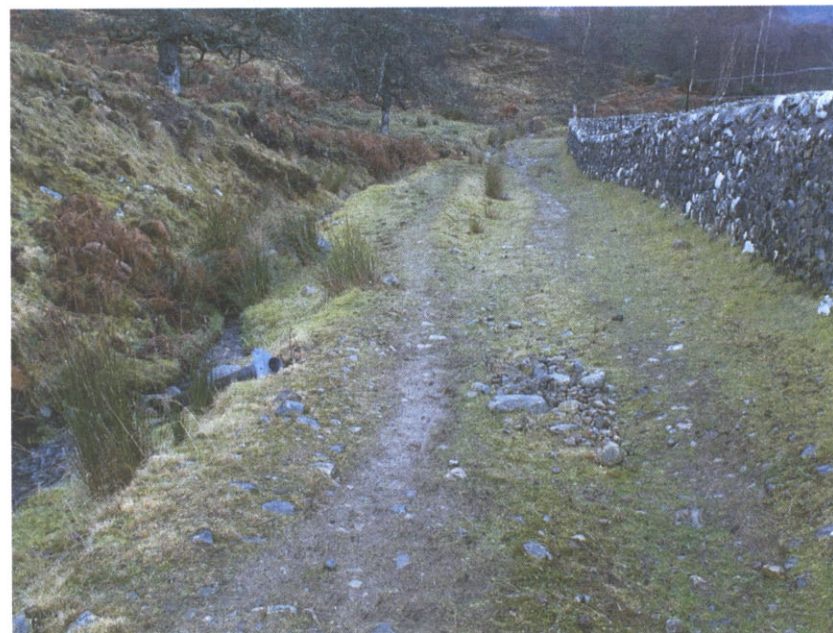
CH350 – Rutting on top section
