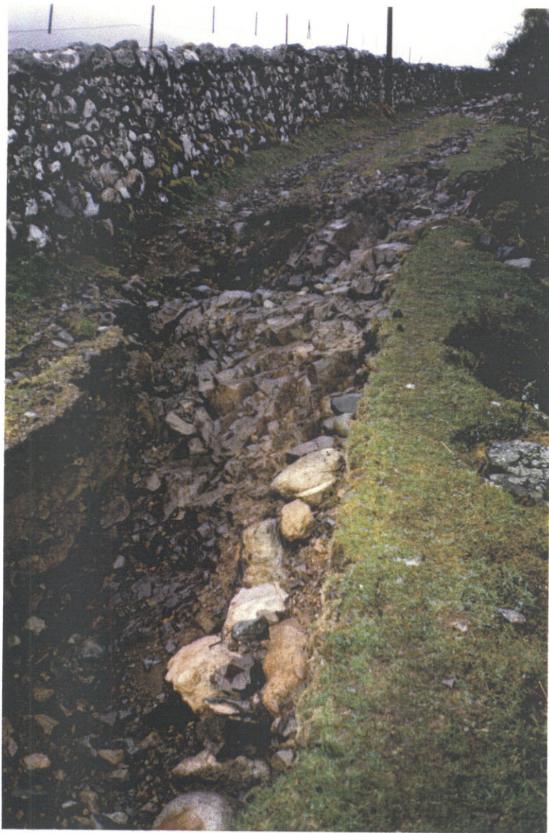
9. Washed out surface, with bedrock and rut, Ch. 210. Sides of ditch collapsed.
