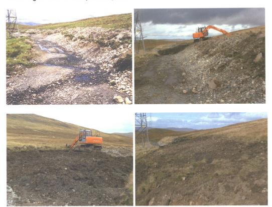
B-NN 40331/99505 - existing access point used in July 2002 for Optic cable works with burrow pit. Burrow pit landscaped with material from edge, spot turfed and seeded.
