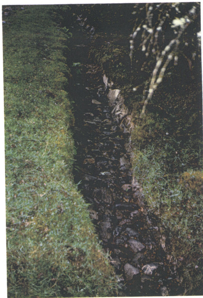
4. Paved ditch in good condition. Ch. 90
