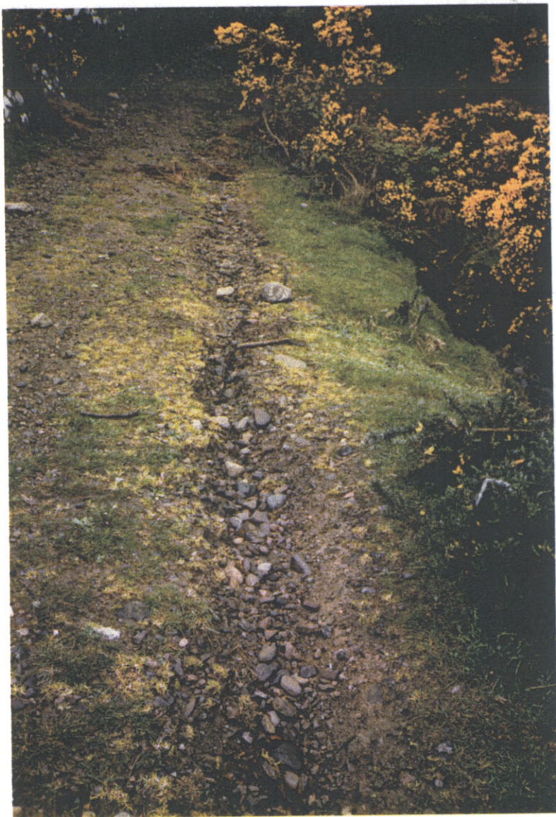
3. Existing road surface with minor rutting. Ch 70
