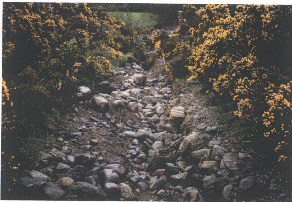
1. Looking downhill to public road. Showing road surface washed away and start of deep ruts.
