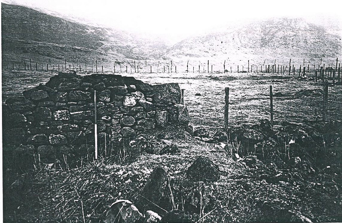
Fig 12(ii) Filled-in cruck slot to right of ranging rod in North wall of building at Site 12. Note possible turf walling on top of stone wall.
