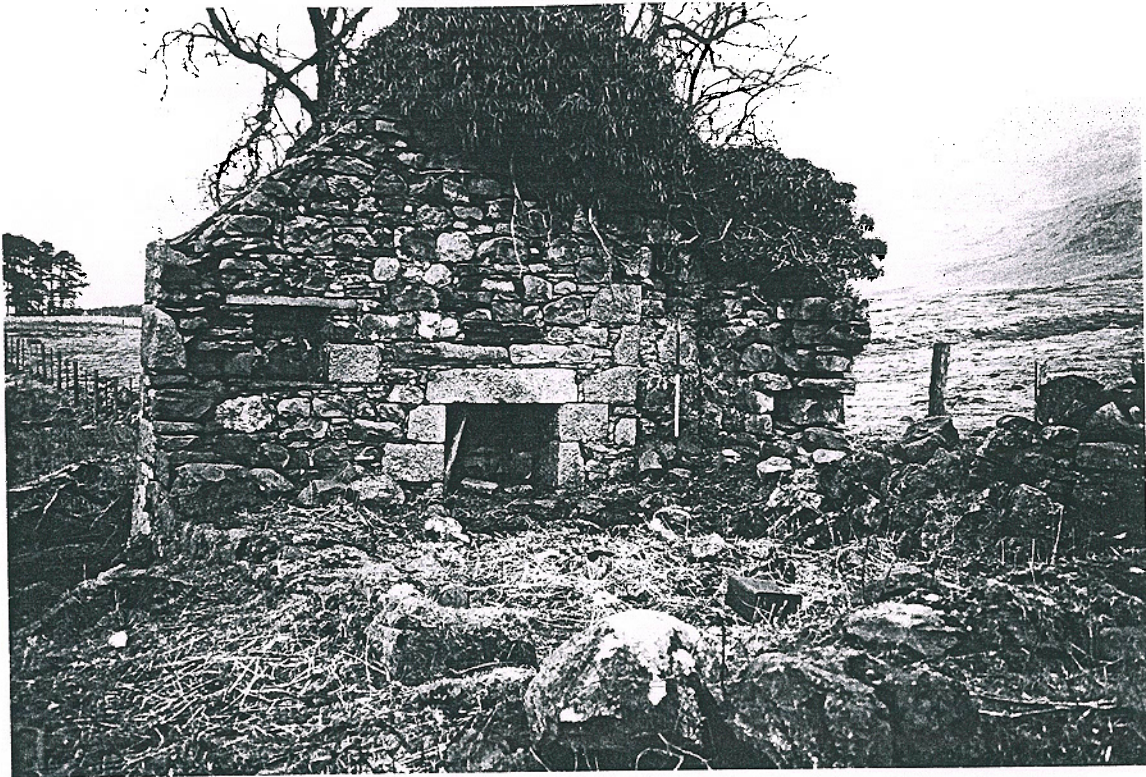
Fig 12(i) Former cruck-framed house showing where gable and chimney has been added Looking West.
